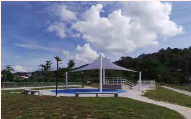
Centrestage of the BECO Park.
